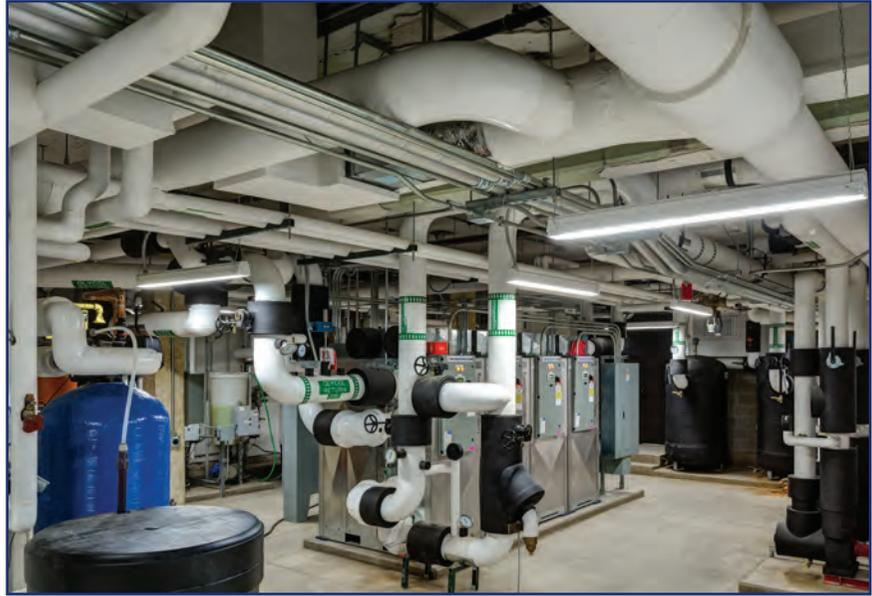
The heart of the mechanical system is a four-module geothermal heat pump system, generating both heating water and chilled water. The geothermal system consists of 56 vertical bore wells, totaling more than 8.5 miles of below grade piping.
