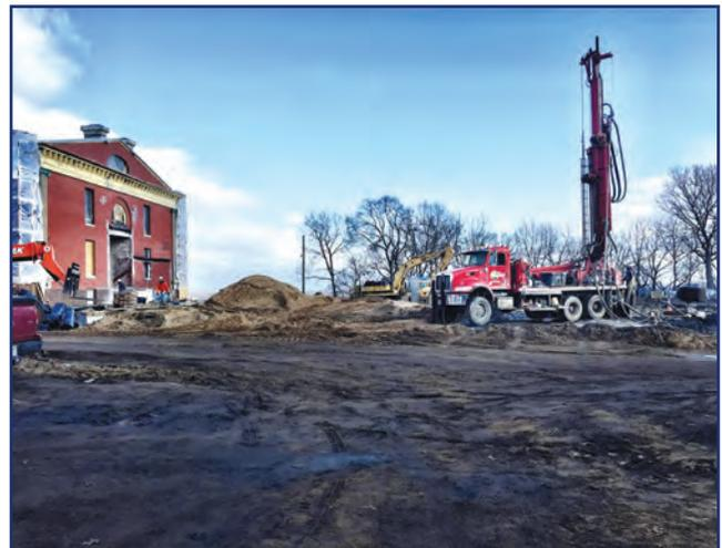
Fifty-six vertical bore wells were installed beneath the parking lot. The well field is designed for future expansion to pick up additional buildings around the site.
